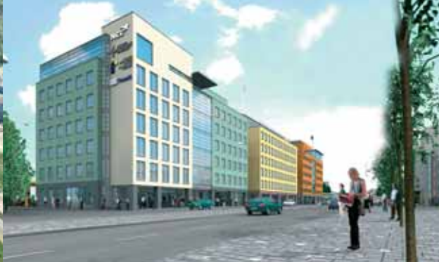
NCC Building 3, Helsinki
